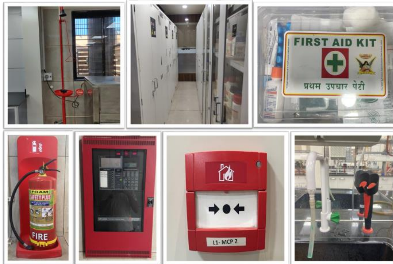
Emergency Eye Washer and Safety Shower
