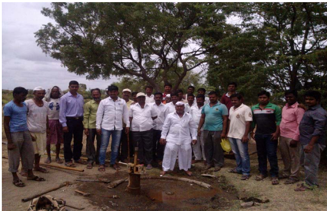
Installation of Hand pump designed by ICT, at Aatpadi Village, Dist. Sangali, Maharashtra.
