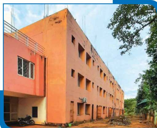
ICT IOC, ODISHA CAMPUS, BHUBANESWAR
