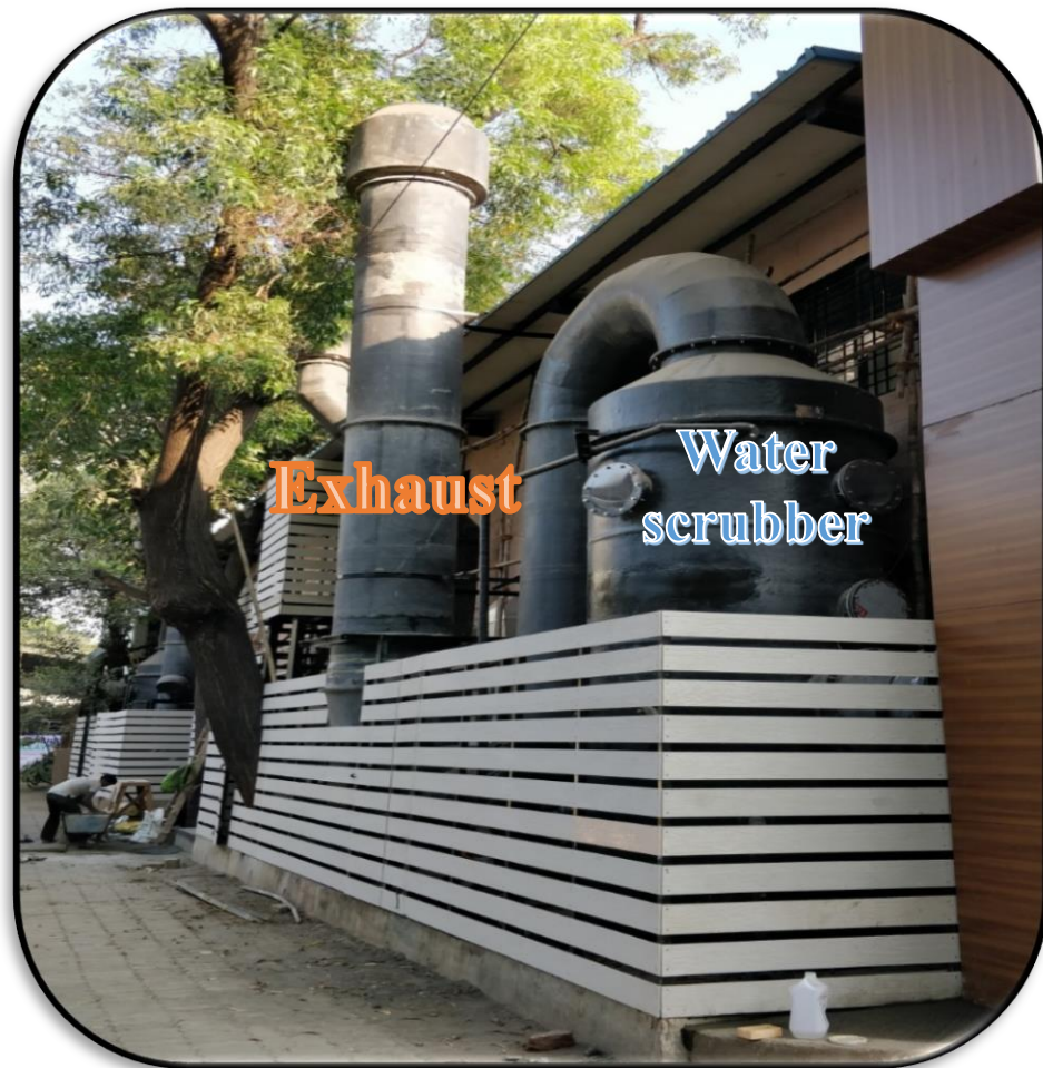
Department of Speciality Chemicals Back View
